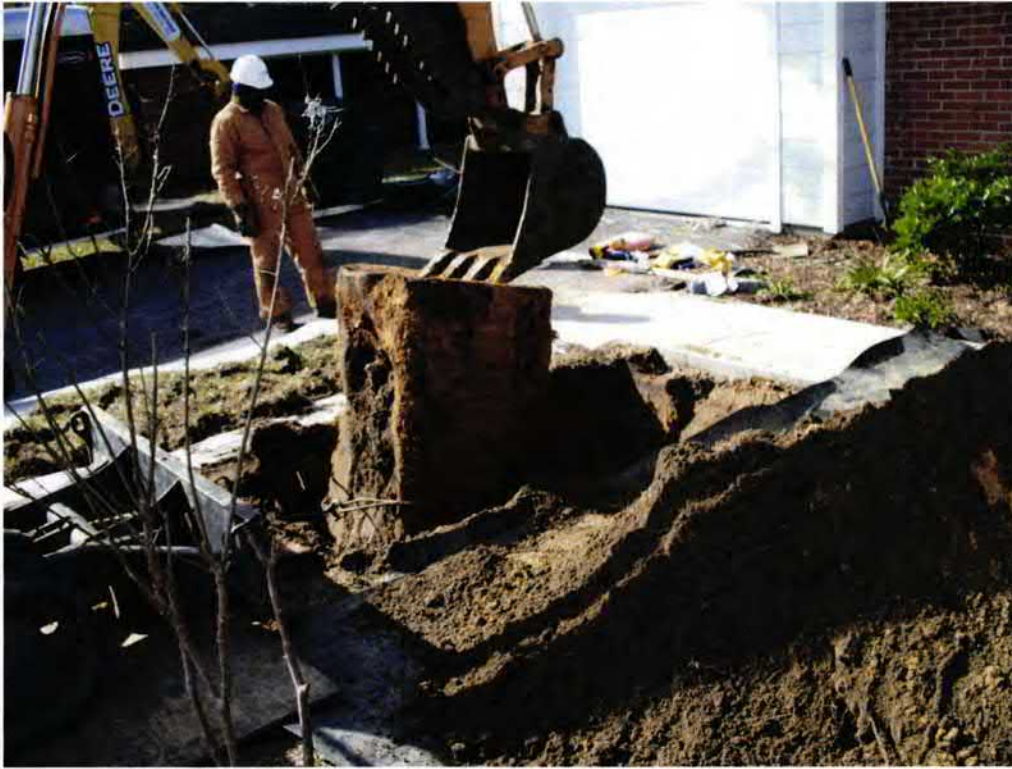
Picture 3: UST 622Dahlia-2 being removed from the excavation.
